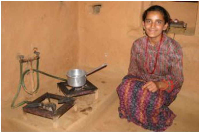
A biogas plant provides clean gas for cooking (BSP, Nepal – photo credit Martin Wright)
