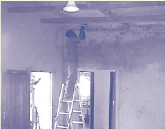
Technician carrying out internal wiring – ladders form part of the tools that they have to carry around. (Photo: Courtesy of Nuon-RAPS Utility Pvt. Ltd.)
